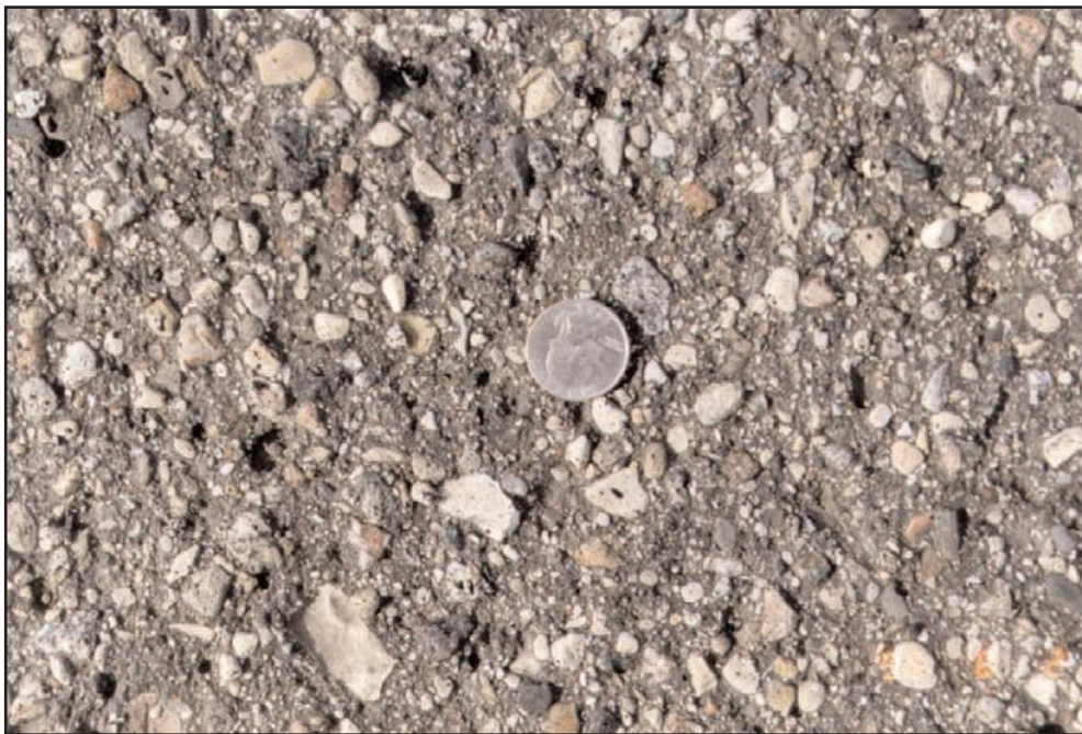
Figure 3.4.10. Example of a highly pocked, porous, and oxidized surface
