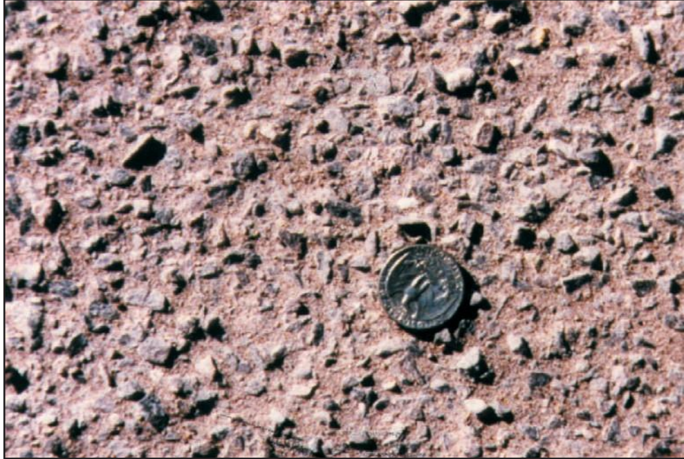
Figure 3.2.10. Dusty aggregate after sweeping (notice most of the large aggregate is missing)
