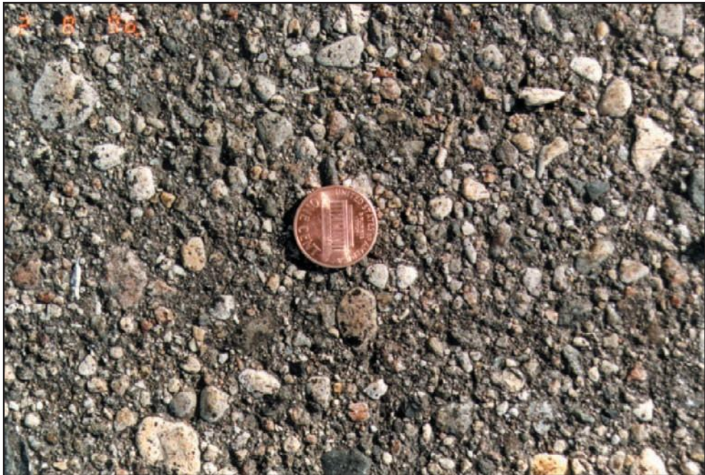
Figure 3.4.8. Example of a slightly porous and oxidized surface
