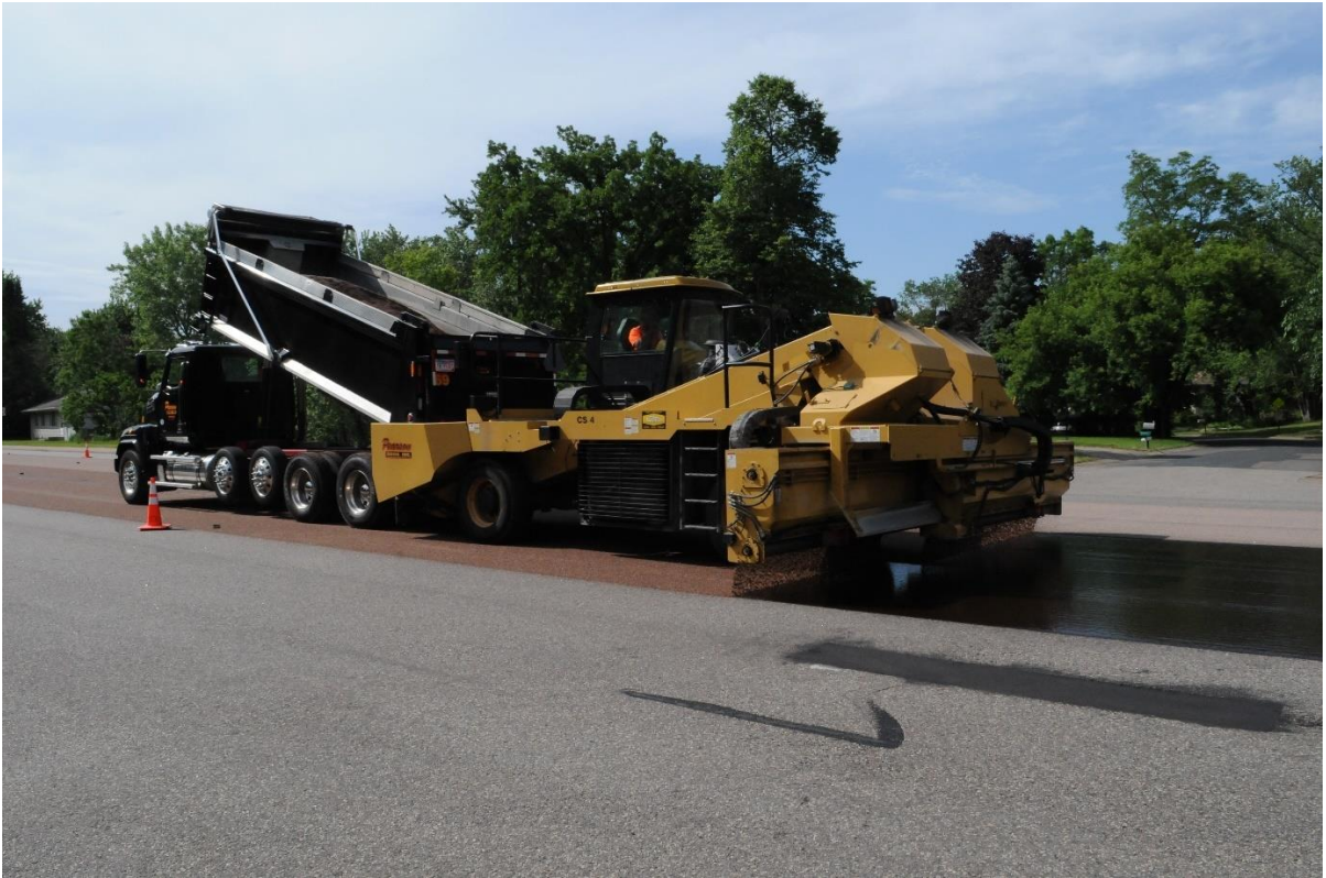
Figure 3.1.7. Self-propelled chip spreader
