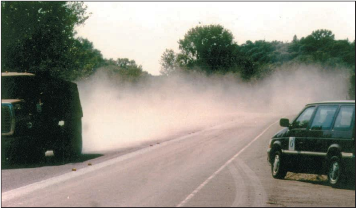
Figure 3.9.6. Evidence of a dusty aggregate
