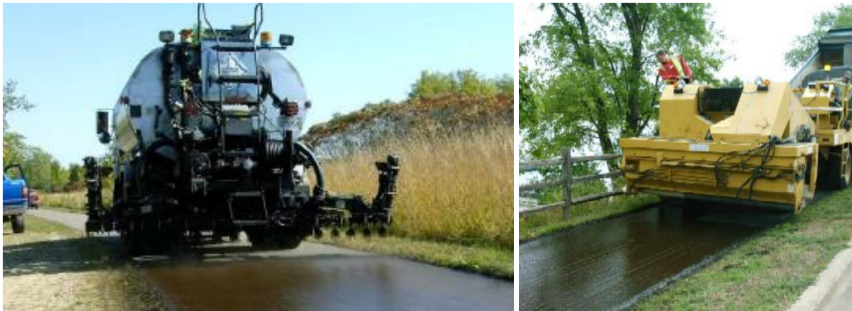
Figure 3.6.1. Chip sealing of recreational trail
