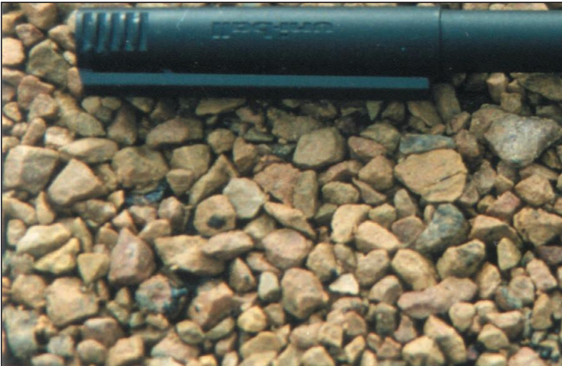
Figure 3.7.2. Too much aggregate (no binder is visible)
