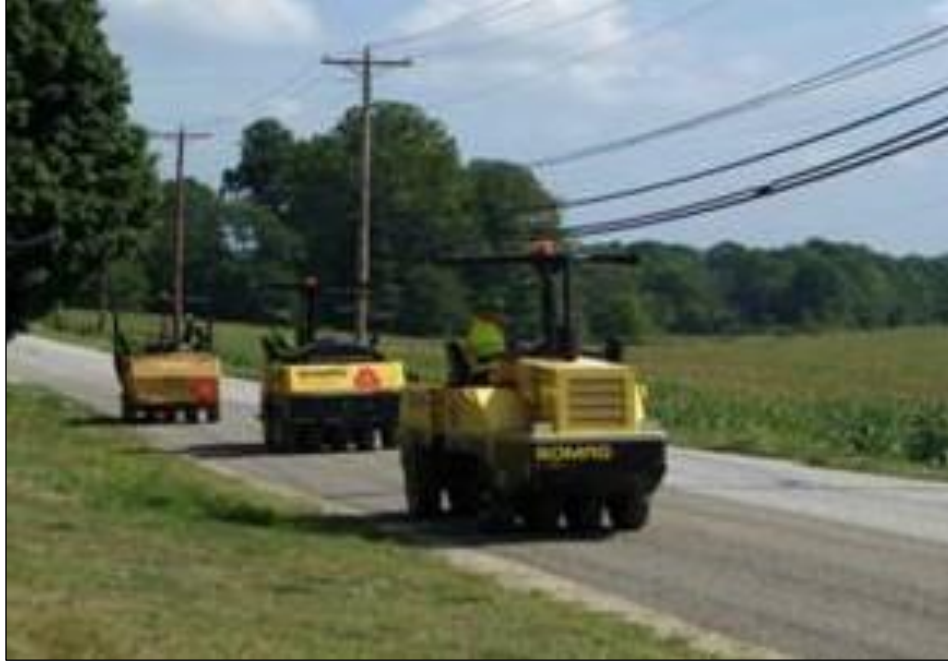
Figure 3.1.8. Pneumatic tired rollers (Ohio DOT)
