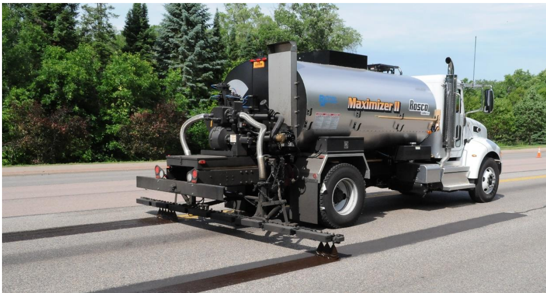
Fig. 3.7.1. Pretreatment of pavement markings prior to chip seal (MnDOT - Paul Nolan)
