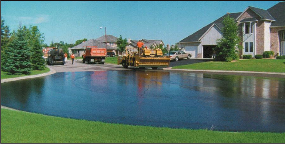
Figure 3.8.22. Wrong way to sealcoat a cul-de-sac (emulsion will break before chips are placed and rolled)
