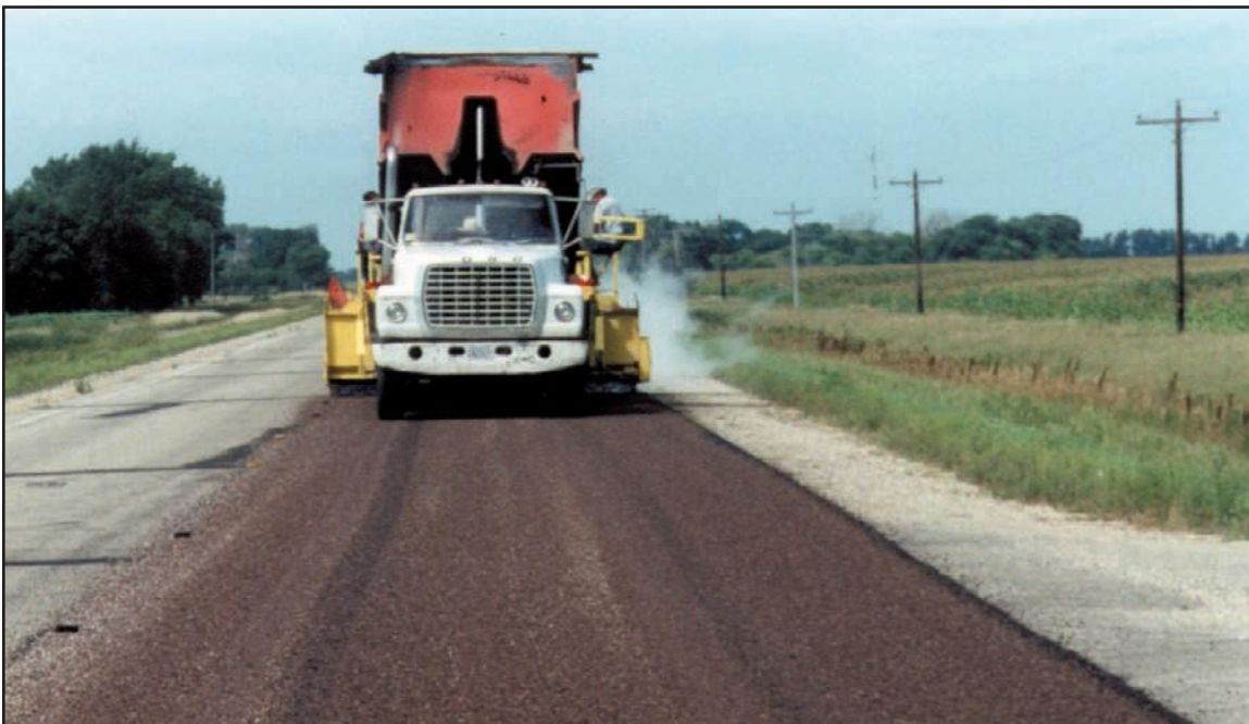
Figure 3.7.5. Darker wheel paths indicate binder has risen near the top of the aggregate
