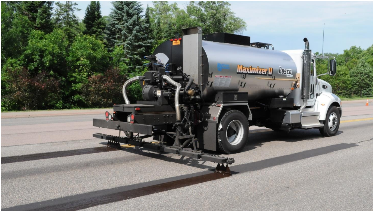
Figure 3.8.21. Pretreatment of pavement markings
