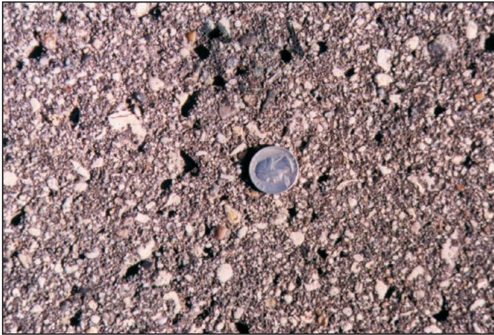
Figure 3.4.9. Example of a slightly pocked, porous, and oxidized surface
