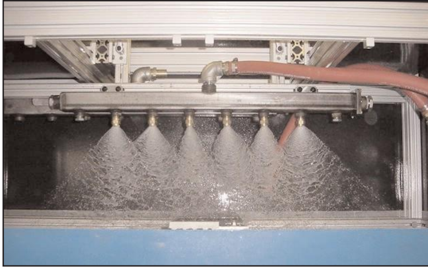
Figure 3.8.7. Spray bar nozzle showing poor alignment
