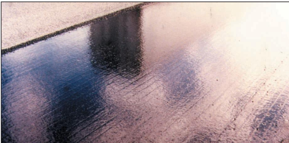
Figure 3.9.4. Example of streaking caused by incorrect spray bar height (notice streaks)
