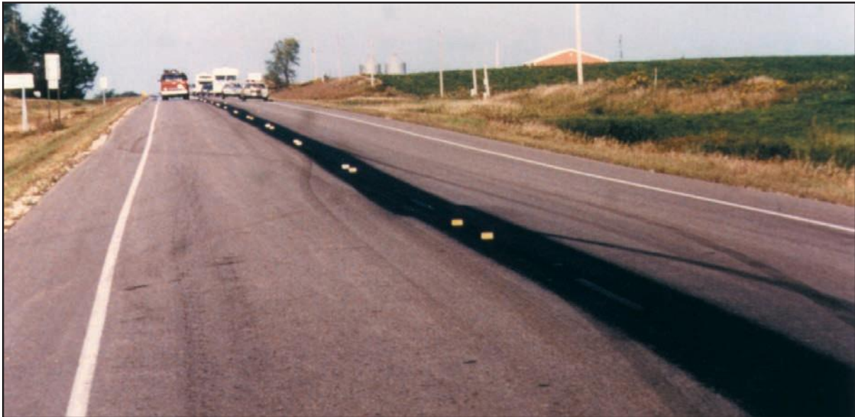
Figure 3.9.7. Fog seal on centerline prior to chip seal to prevent excess absorption
