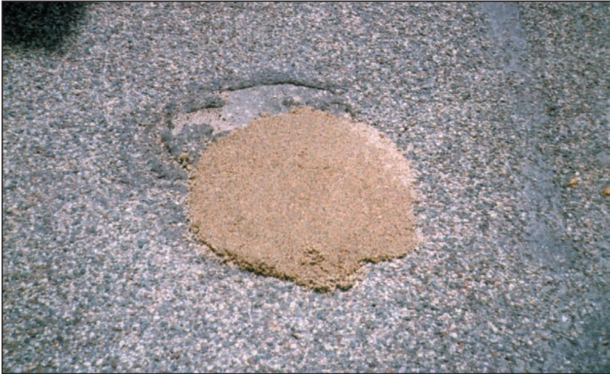
Figure 3.8.23. Sand cover on manholes
