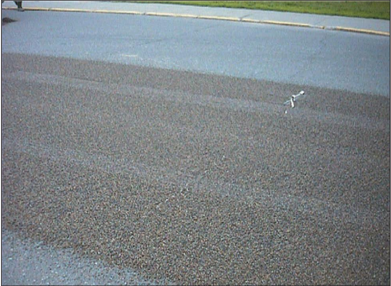
Figure 3.8.2. The rubber mats are covered with aggregate from the chip spreader
