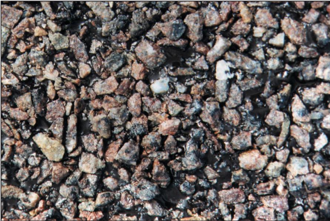
Figure 3.7.4. Correct amount of binder (binder has risen to top of chips)
