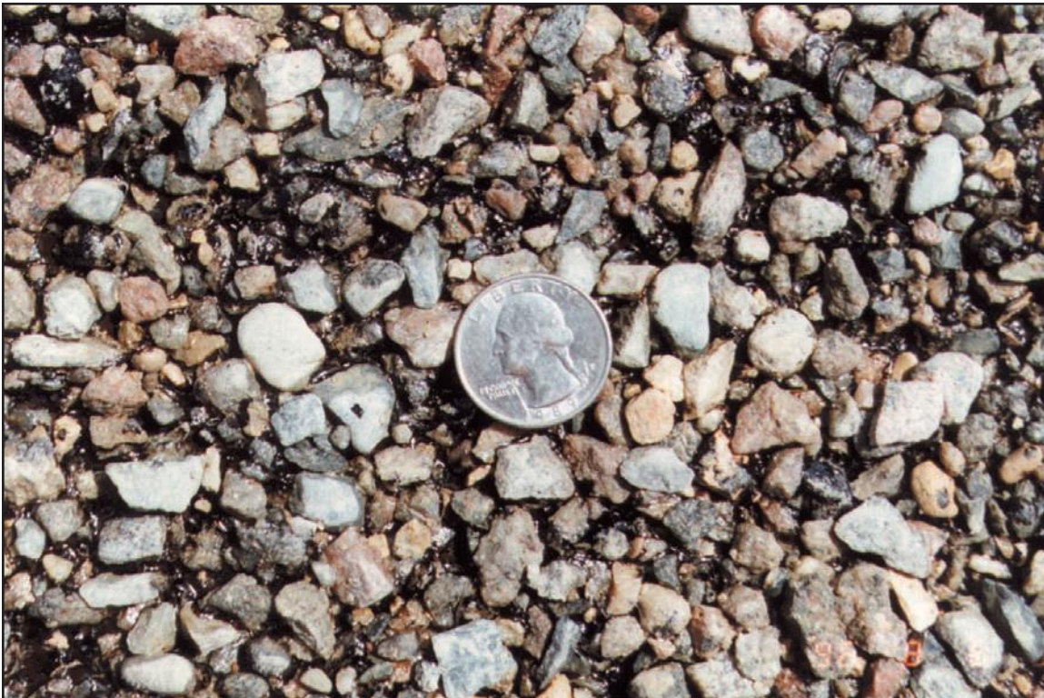
Figure 3.7.3. Not enough binder (binder is too low)
