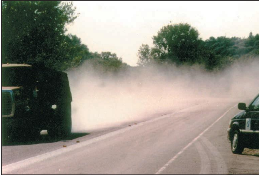
Figure 3.2.8. Evidence of a dusty aggregate
